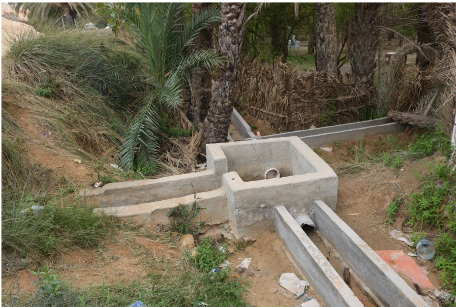
The irrigation water is brought to the plots through these cemented canals. (photo: Myrah Vandermeulen)
